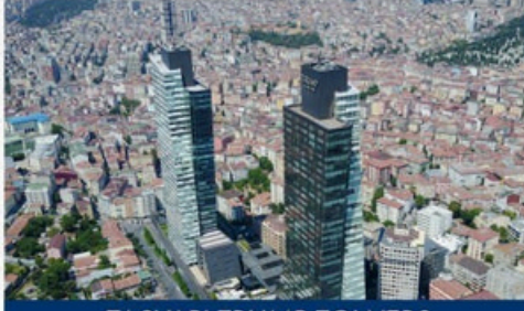
TAŞYAPI TRUMP TOWERS
